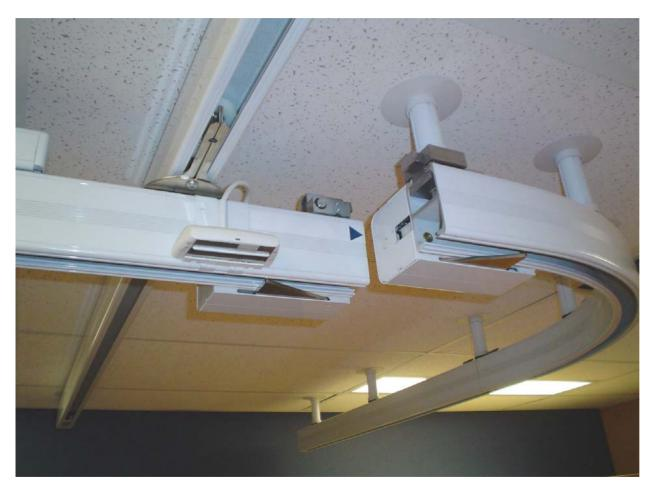
A Gate allows you to travel the lift from an XY System to either straight or curved tracking to gain access into washrooms or other rooms.
