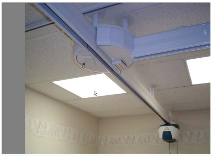
A turntable allows you to join many tracks running in different directions together in one junction.
