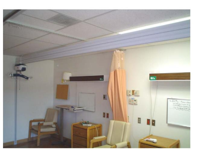
Wall to Wall install using wall posts. This is necessary when installation into the ceiling is not possible.
