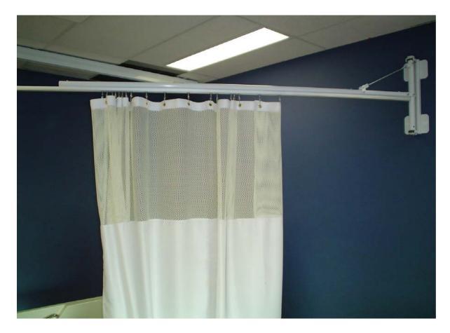
A pivoting curtain rod allows you to drop the privacy curtain underneath the tracking in order to eliminate any interference with the lift.
