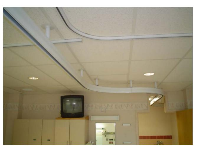
Curved Track installed through door header and into washroom. Due to the difference in height from the ceiling in both areas the tracking was dropped to accommodate the lower of the two ceiling heights
