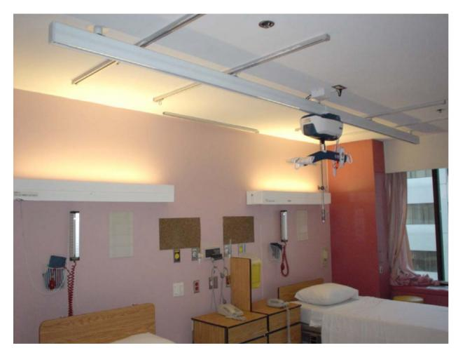
Straight track installed in Semi-Private room with concrete ceiling. This is accomplished using powder coated exposed uni-strut.
