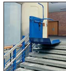
Inclined platform lifts
